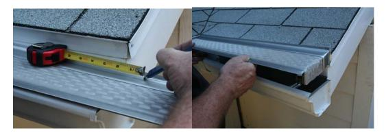
**Step 4**, Optional screws may be utilized at the sight line channel into the fascia to provide additional structural support for the entire gutter system.
