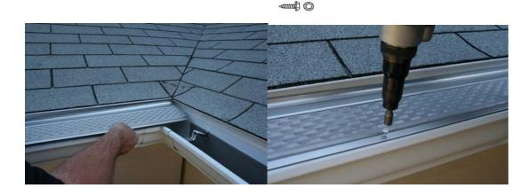
**Step 2.** When reaching the gutter corner, mark and cut a diagonal angle beginning from the gutter nose. Begin the **Clean-Mesh** panel angle cut at the front lip, then snip the weep hole leg, and begin the angle cut at the gutter systems back corner and cut towards the front of the panel. Cut and remove the face of the next **Clean-Mesh** panel to conform to the angle and butt tight together.
