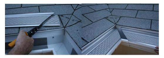
**Step 3.** At the termination end of the gutter system, you will need to snip and remove the panel nose and the weep hole leg approximately 2" from the gutter end. Bend the 2" section downward at a 90 degree angle to create a cap at the end of the system. This will prevent debris and pest from interring the gutter system at the end
